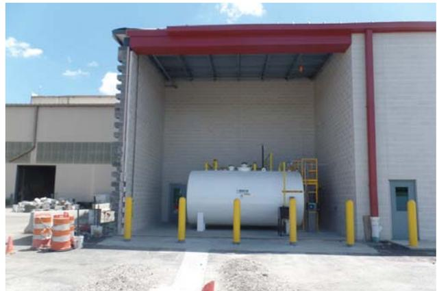
*Pictured above is a 6,000 gallon auxiliary #2 diesel fuel tank used to fuel equipment at the Resource Recovery Center.*
